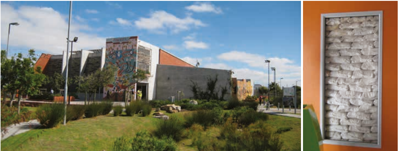
Figure 4. Photo of the Manenberg Human Settlement Contact Centre’s main façade – on the left – and of the “eco-beam & sand technology” used – on the right.
