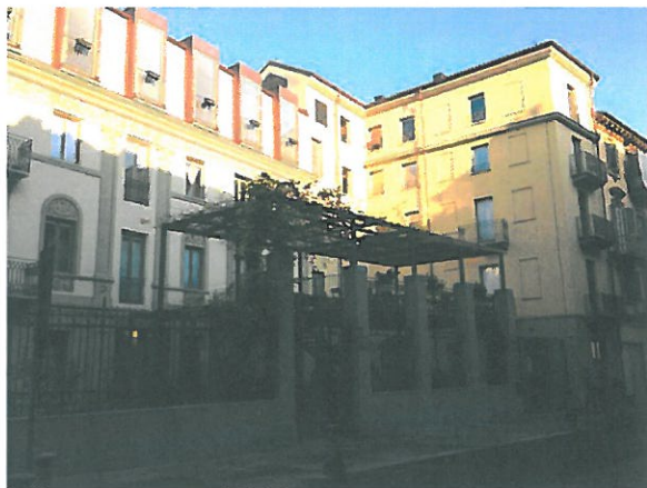
Fig. 2 San Salvario Temporary Residence.
