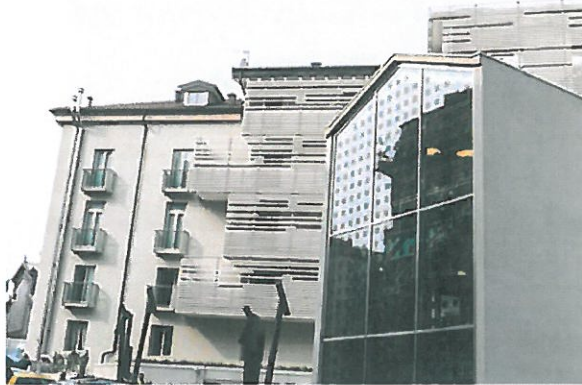
Fig. 1 Porta Palazzo Temporary Residence.
