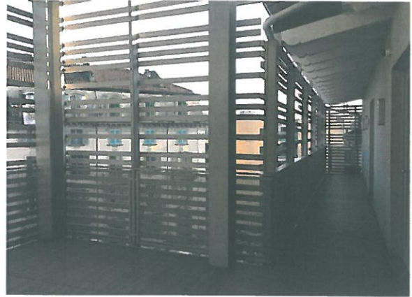
Fig. 10 Distribution corridor to the living units.
