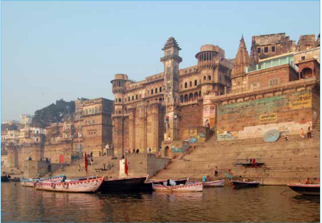
Fig. 3 - Varanasi, Darbhanga Ghat. The architectural and historical heritage is surrounded by the river and by new less historical structures.
