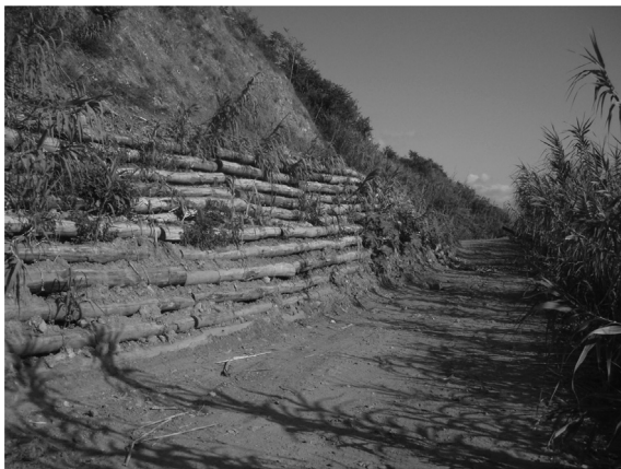
Fig. 6. View of the Fuscaldo (Cosenza) installation on the mountainside along a road. Elements of the structure were installed on two alignments one upon the other (Barbero et al., 2013).
