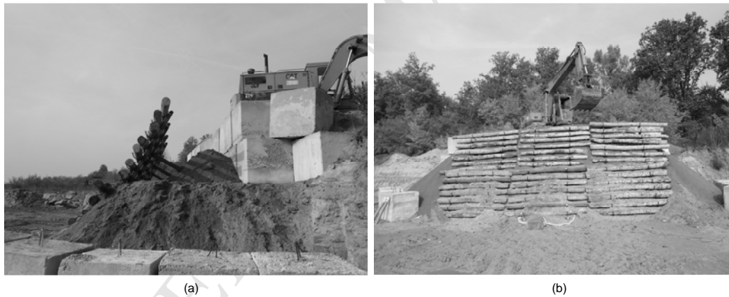
Fig. 5. (a) Filling phase and (b) placing of the upper alignments.
