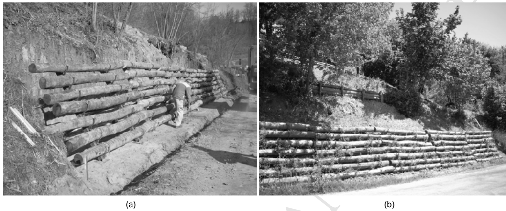
Fig. 4. Example of the structure installed at Roatto (Asti, Italy): (a) the element before the filling, and (b) final configuration when the bushes start growing.
