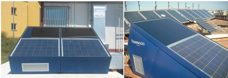
Fig. 1. Freescocoo compact prototypes installed at ENEA in Rome (left) and at UNIPA in Palermo (right)
