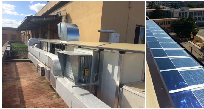
Fig. 2. Desiccant AHU based on the freescoc concept
