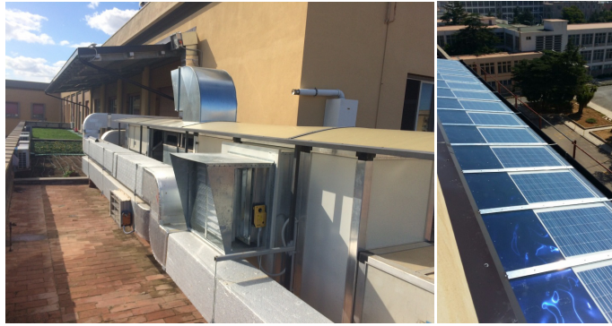
Fig. 2. Desiccant AHU based on the freescoc concept
