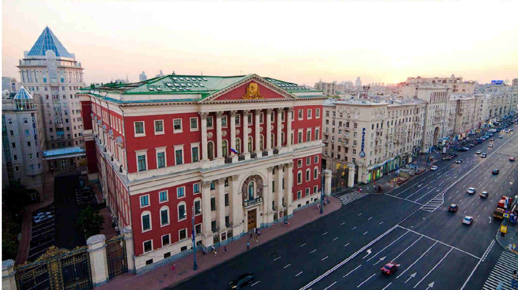
Fig. 4 - Chernyshev House, project by M.Kazakov. Now it is the building of the Moscow mayor's office.
