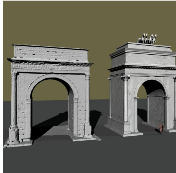
Figure 12. Reconstructed model of the Arch of Augustus: on the left the laser survey model; on the right the model inspired by Cesare Bertea and Luigi Rossini's studies (Mercando, 1993).
