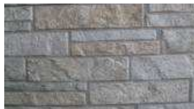
Fig. 34/35/36- Facades' details. Cladding in plastic- Kamisaginomiya - Tokyo. (Photo by the Author)
