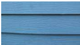
Fig. 34/35/36- Facades' details. Cladding in plastic- Kamisaginomiya - Tokyo. (Photo by the Author)
