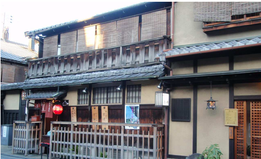
Fig. 7 – Kyoto - Facades in Gion Area. (Photo by the Author)
