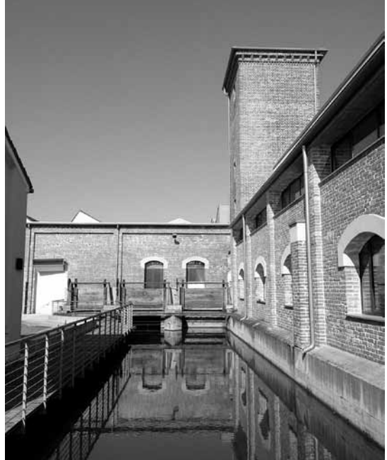
Figure 3.1. An example of a successful brownfield reconversion with economic and social feedback in a small town in Italy - Ex Jutificio in Piazzola sul Brenta (Padova) (Dragotto, 2012).
