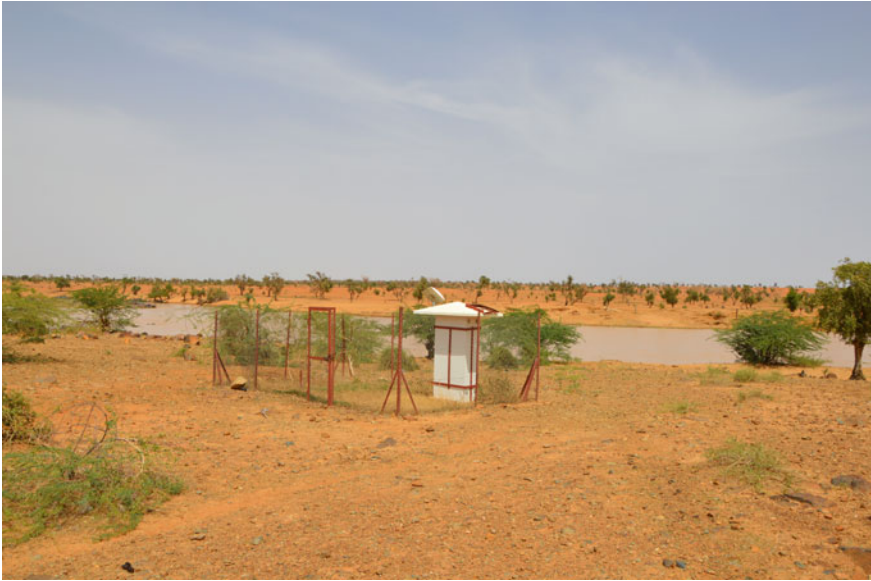
Fig. 11.4 The Sirba hydro station at Garbey Kourou in June 2014
