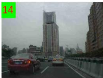
14 Yan'an Elevated road
