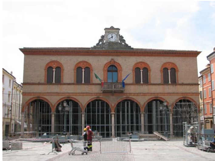
Fig. 1 Mirandola Town Hall after temporary safety measures
