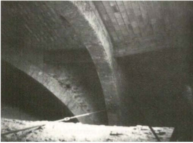
Figure 7- Tie installed during the 1958 (Rocchi, 2002).
