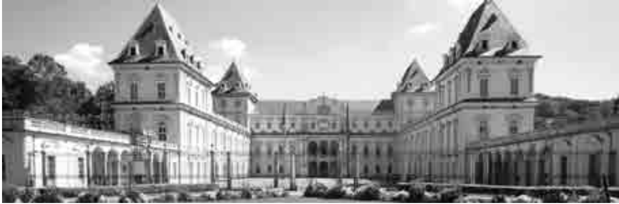
Figure 1. The case study: photography of the main building of Valentino Castle.
