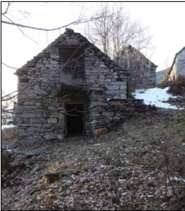
Figure 2. Typical Alpine stone building
