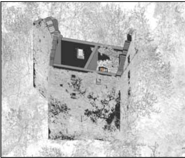
Figure 5. Creation of a parametric 3d model of the castle from the laser scanner point cloud (Osello, E., 2012)
