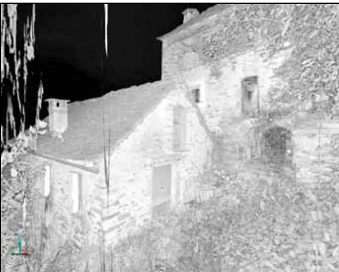
Fig. 3. Laser scanner 3D survey of a traditional Alpine stone building
