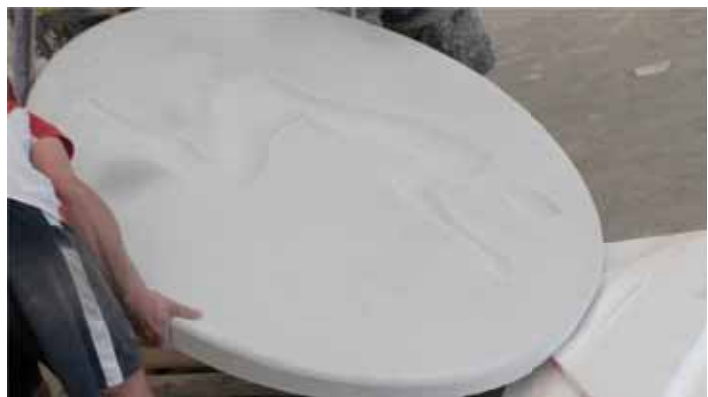
Fig.7. Public artwork 'Identity'. Form stripping to 48 hours after casting (Company Paolino Ciabrone).
