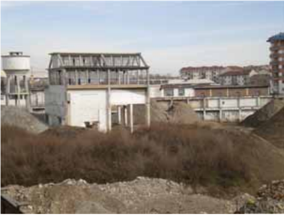
Fig. 1. Area of Spine 4 Park, Turin, at the start of reclamation, in February 2010.
