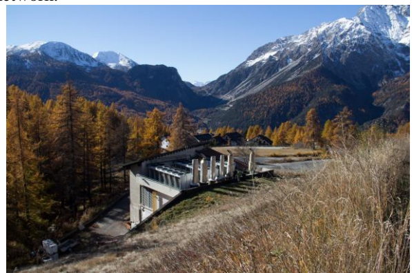
Figure 2 – Cogeneration Station and surroundings
