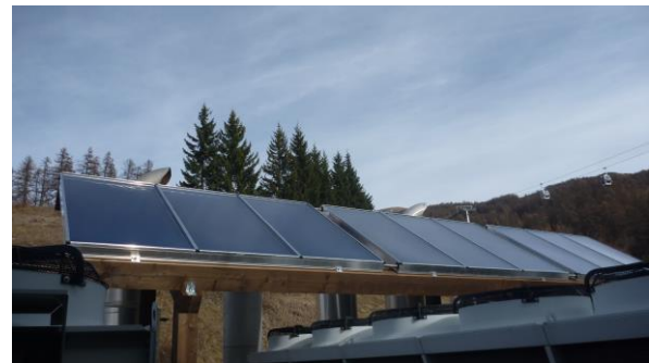
Figure 4 – FPC installed
