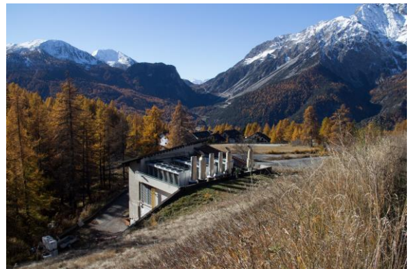
Figure 2 – Cogeneration Station and surroundings
