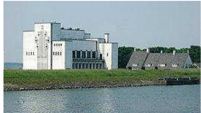
Dirk Roosendaal, Electrical pumping station for the Wieringermeerpolder, 1928–30
