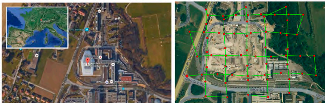
Figure 3. The case study: EFPL's SwissTech Convention Center in Lausanne, Switzerland. In the right image there is an example of the flight plan and image acquisition.
