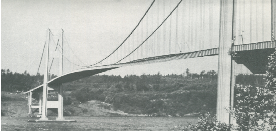
FIGURE 1. The collapsed Tacoma Narrows Bridge (1940).
