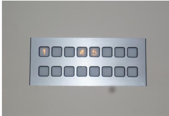
Figure 9.3. Example of assistance request mechanism within a RAF2 bathroom. Here the panel indicates who is requesting assistance.
