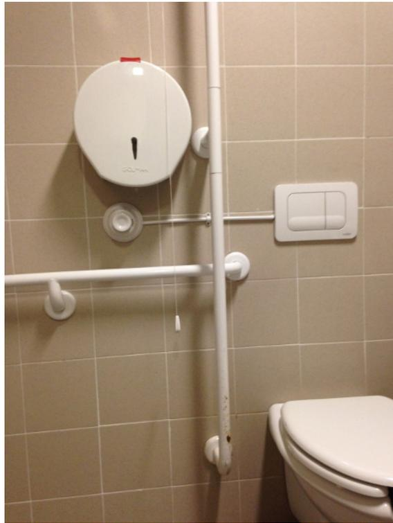
Figure 9.2. Example of assistance request mechanism within a RAF2 bathroom. Here the buzzer is operated by pulling a string.
