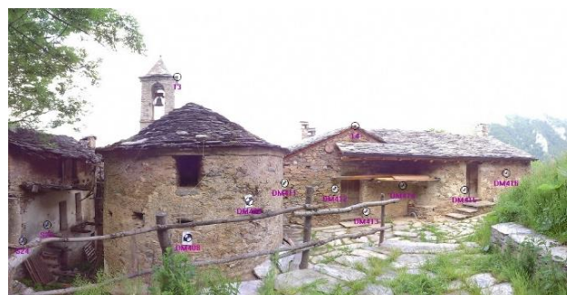
Figure 4. The use of measured targets for the registration phase.
