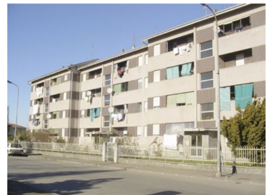
Figure 2. Social housing settlement before and after renovation.
