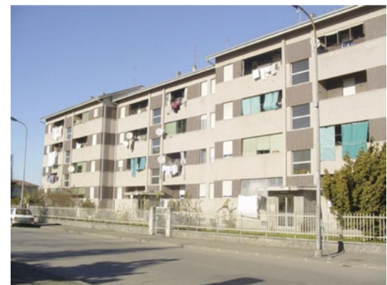
Figure 2. Social housing settlement before and after renovation.
