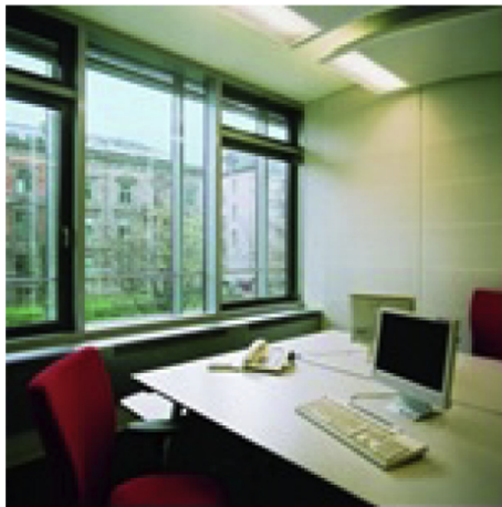
Fig. 3. Offices with operable windows and sun protection, allowing natural ventilation and natural lighting.
