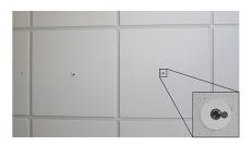
Figure 4.17: Ultrasonic receivers in ceiling tiles
