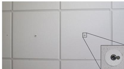
Figure 4.17: Ultrasonic receivers in ceiling tiles
