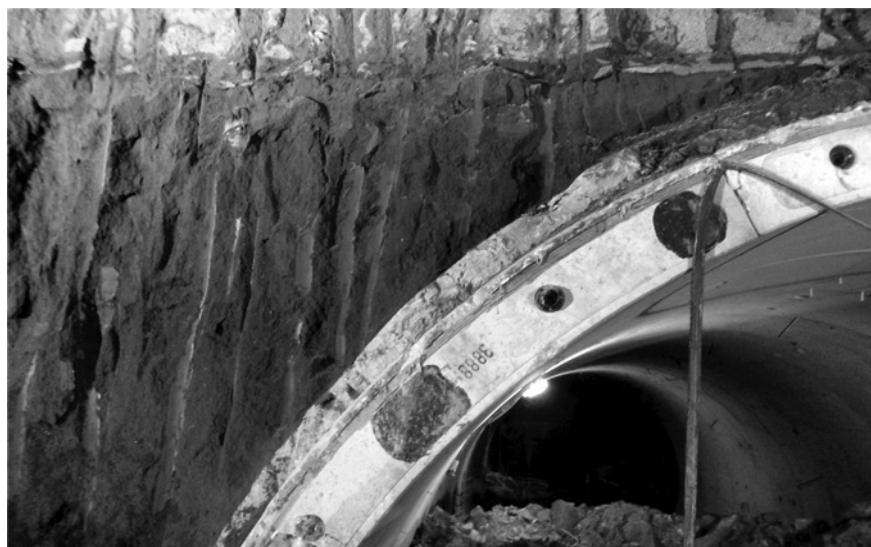
Fig. 2. Hardened two component mix below the segments and the soil as shown in the excavation of the station Centocelle. (photo Mapei's archive).
