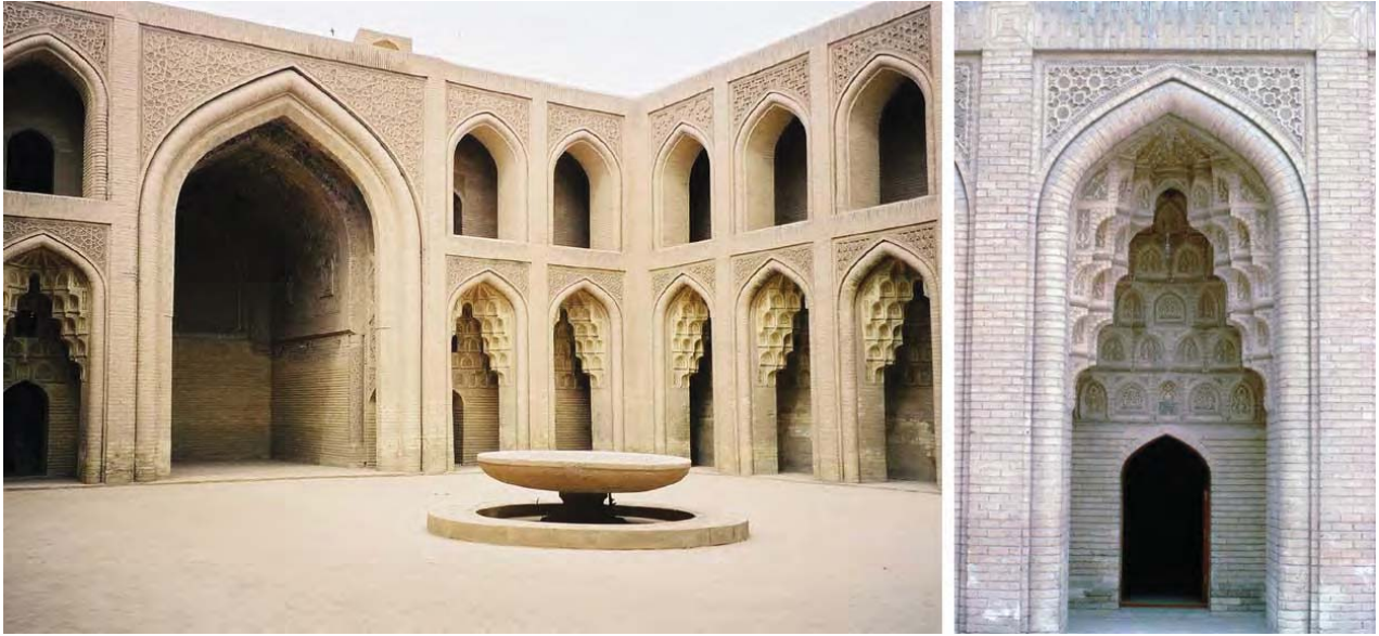
Fig. 6: Detail of the decoration of the madrasa of Qal'a in Baghdad (XIII century). Pulling back the bricks arranged in horizontal than vertical generates a pattern in slight relief emphasized by square terracotta stamped.
