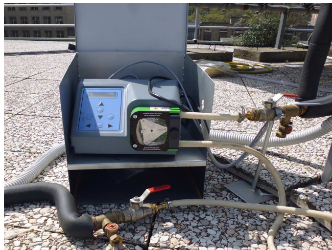
Figure 7 Full scale prototype: peristaltic pump.
