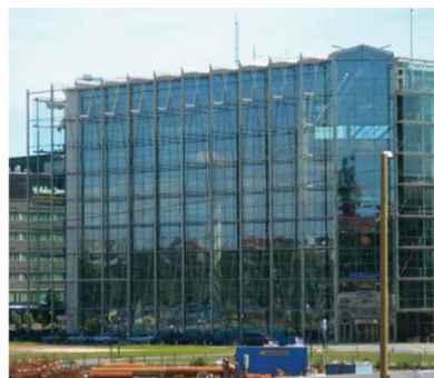
Helsinki - Finland T_{\text{design, winter}} \approx -24 \text{ }^{\circ}\text{C} \text{HDD} \approx 4786 \text{ }^{\circ}\text{C}\cdot\text{d} T_{\text{design, summer}} \approx 25 \text{ }^{\circ}\text{C}
