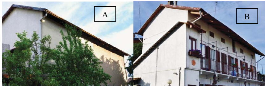
Fig. 1. Typical example of building envelope optimization in traditional architecture, based on the classical approach of the ‘energy conservation’ – HDD = 2894°C · d, winter design temperature –8°C, summer design temperature 32°C, CDD = 386°C · d – (ASHRAE, 2013) (A: north exposition; B: south exposition).
