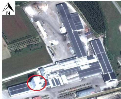
Fig. 2. Satellite image of the 2.5 MWp BIPV system.
