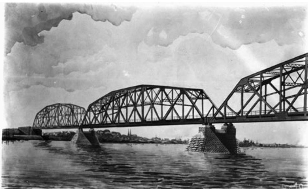
Figure 1: View of the bridge project on the Yellow River, China (1921).
