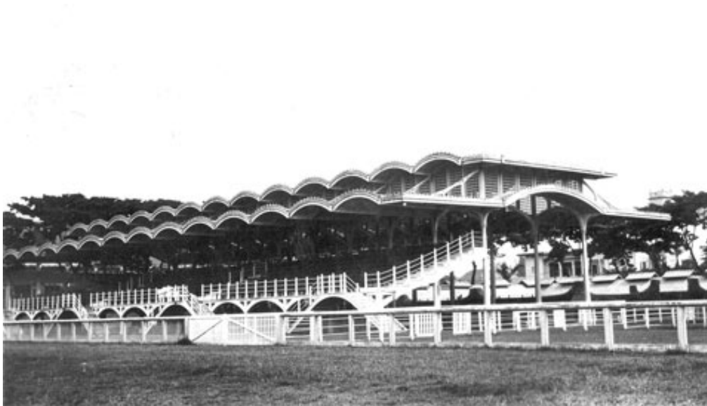
Figure 10: The reinforced concrete seats of the Royal Turf Club in Bangkok, Thailand, designed by the engineer Emilio Giovanni Gollo (1921-2).
