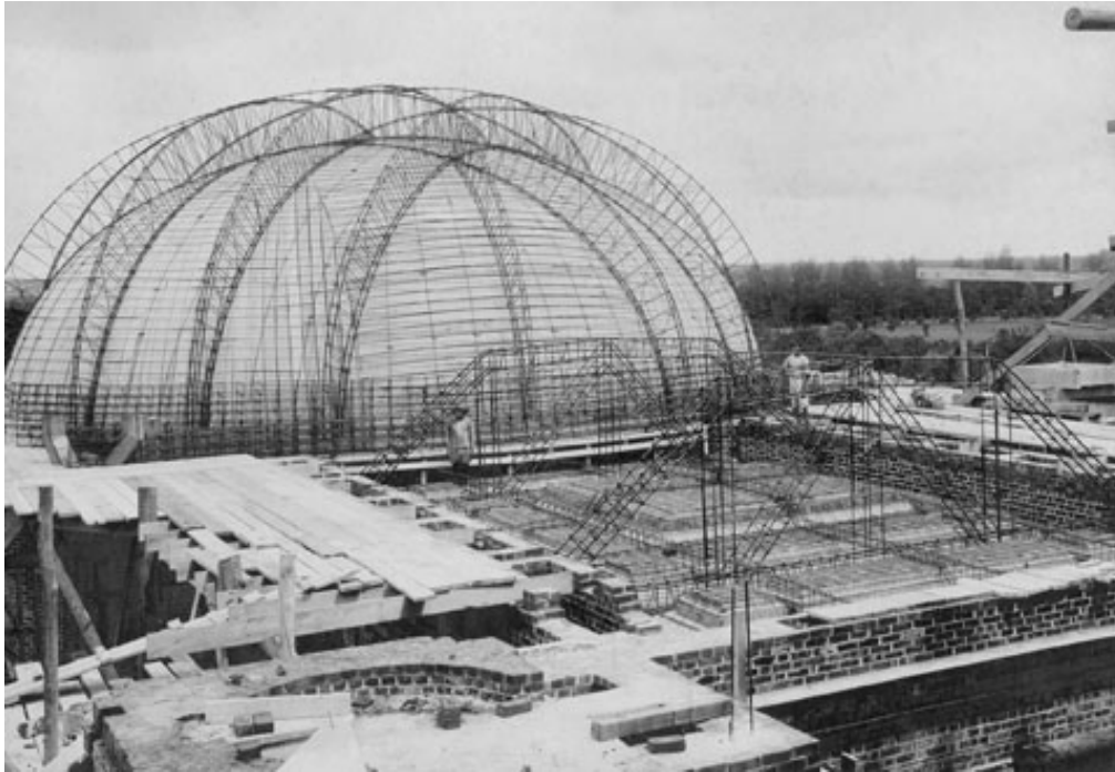
Figure 2: Reinforced concrete works in the Throne Palace building site, about 1911.
