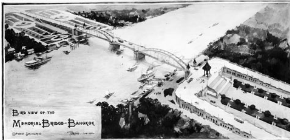
Figure 8: Bird View of the Memorial Bridge at Bangkok, Thailand (1929).
