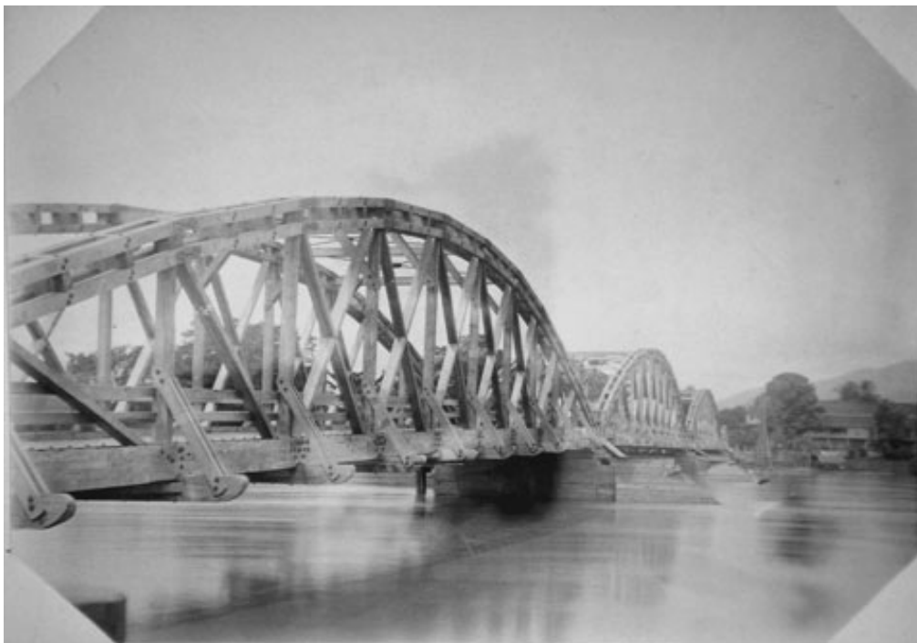
Figure 5: A wooden bridge outside Bangkok, Thailand (not better identified) by the engineer Edmondo Roberti di Castelvero.
