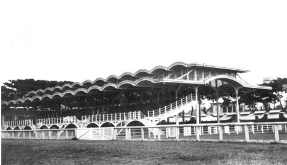
Figure 10: The reinforced concrete seats of the Royal Turf Club in Bangkok, Thailand, designed by the engineer Emilio Giovanni Gollo (1921-2).
