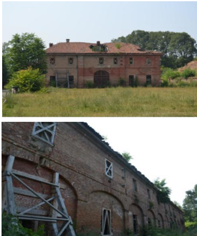
Figure 4 e 5 Front east (left) and North (right) of the building Riding stable Source: campaign photographic survey of Authors (September-October 2013)
