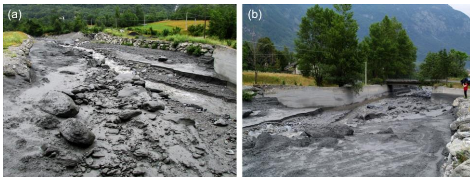
Figure 29 - Detail of the Malo torrent channel bed the day after the debris flow: (a) deposits in the channel bed, photo taken from downstream to upstream; (b) deposits in the channel bed and traces of the passage of the flow on the bridge abutments, view from upstream to downstream (photos taken in the same location where the frames presented in Figure 28 were shot).
