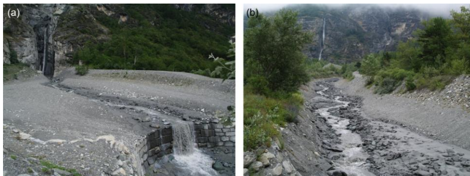
Figure 26 - The waterfall (100 m high) located 376 m upstream the station 1 of the Marderello monitoring station (a) and the monitored reach of the torrent located just downstream the waterfall (b). In these pictures taken on July 18, 2013 is possible to observe the traces of the mud flow that occurred the day before.
