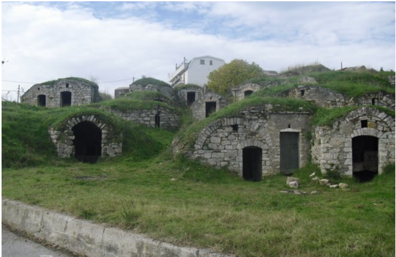
Fig. 8. The "palmenti" in the agrarian territory of Pietragalla, with the modern buildings on the background
