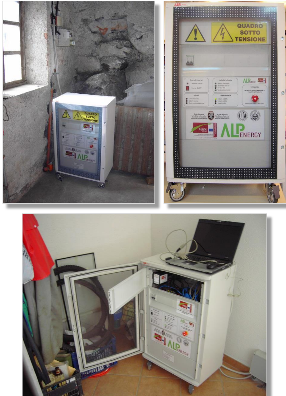
Figure 51: Installation of ESS in citizens houses in Saint Denis
