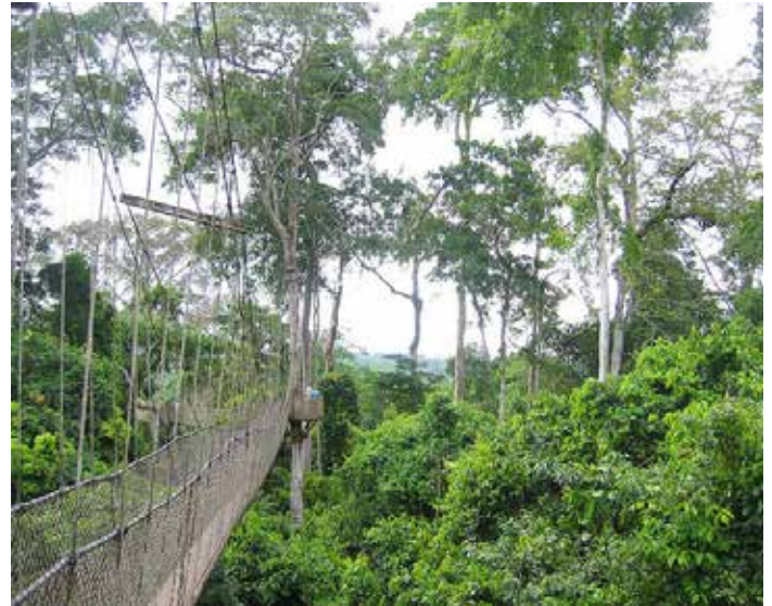
Kakum National Park Canopy Walkway, Ghana (fotografia di Kaylan Neelamraju da www.flickr.com ).
