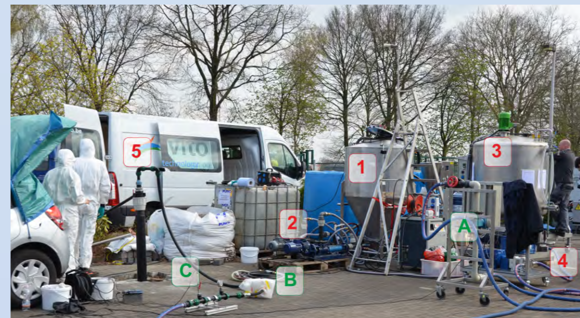
IMZVI field injection at Site P: (1) tank for slurry preparation (2) dispersion and recirculation unit, (3) tank for slurry storage, (4) cation pump, (5) injection well, (A) discharge rate measurement, (B) magnetic susceptibility sensor, (C) pressure sensor.
