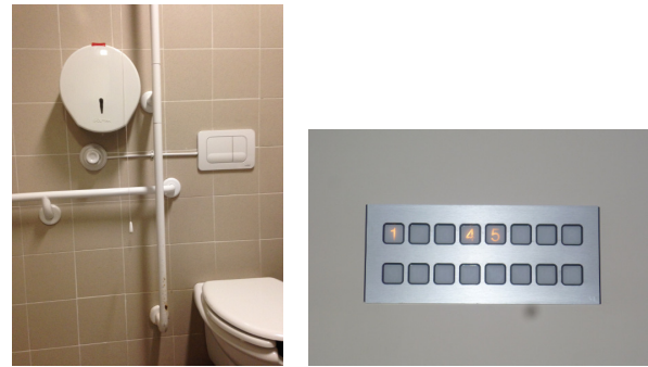
(a) The buzzer is operated by pulling a string (b) The panel indicates who is requesting assistance
