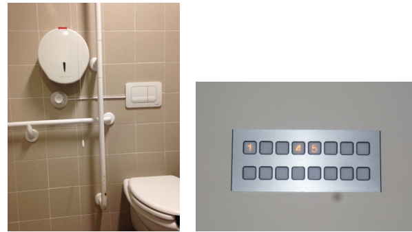
(a) The buzzer is operated by pulling a string (b) The panel indicates who is requesting assistance
