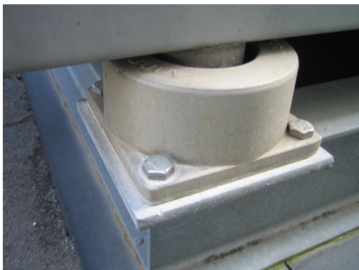
Figure – Vibration eliminator
