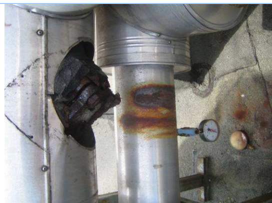
Figure – damaged insulation
