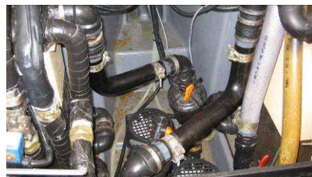
Figure – Li-Cl Solution pumps
