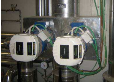
Figure – Pumps with inverter (cool/hot water)
