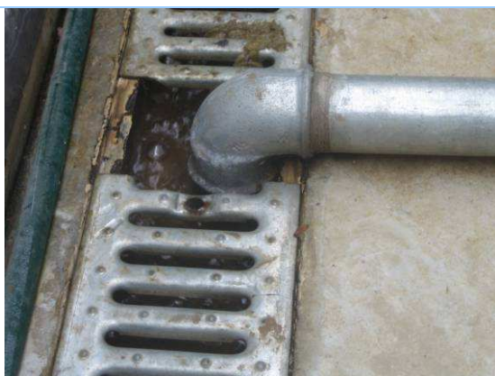
Water discharge due to broke automatic level trigger
