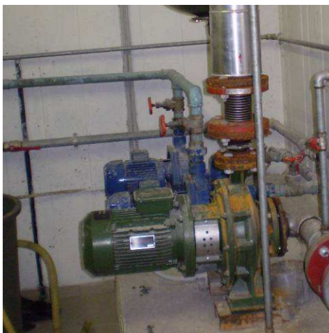
Figure – Well water feeding condenser
