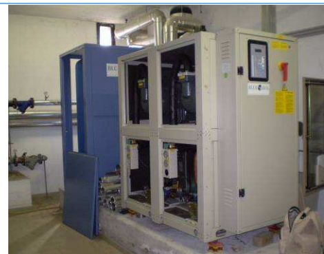
Figure – Cold generator Plant
