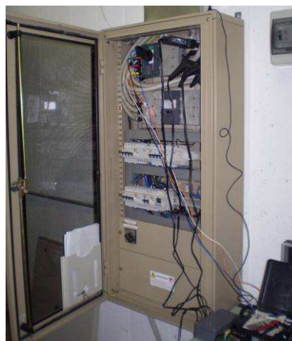
Figure – Electric panel with meter installed
