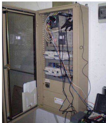
Figure – Electric panel with meter installed
