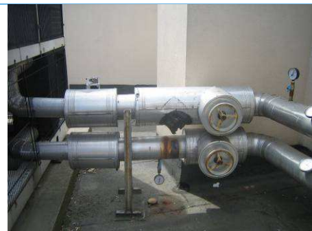
Figure – cool water inlet and outlet
