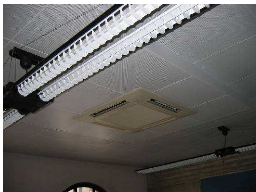
Figure – Internal unit
