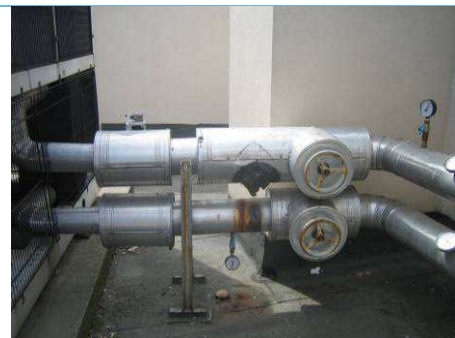
Figure – cool water inlet and outlet
