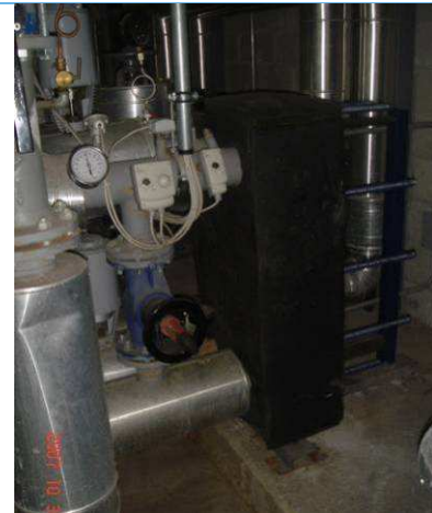
Figure – Heat exchanger
