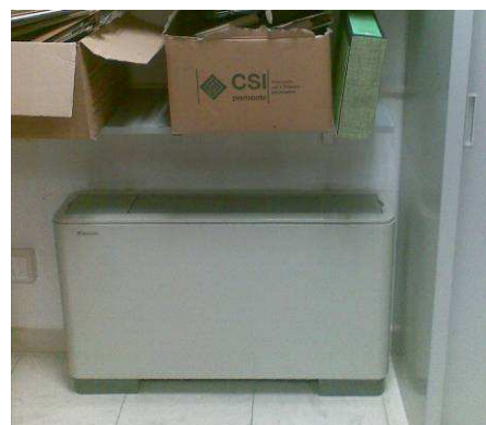
Figure – Internal unit in a inefficient position
