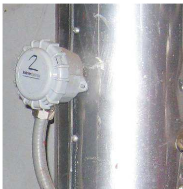
temperature probe on cooling water return
