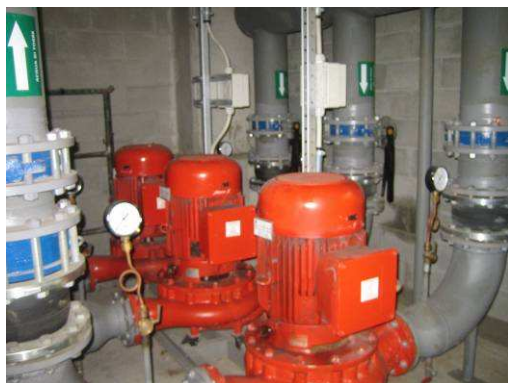
Figure – heat rejection circuit pumping system
