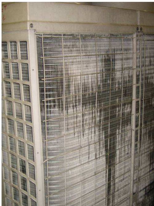
Ice formation on the external units
