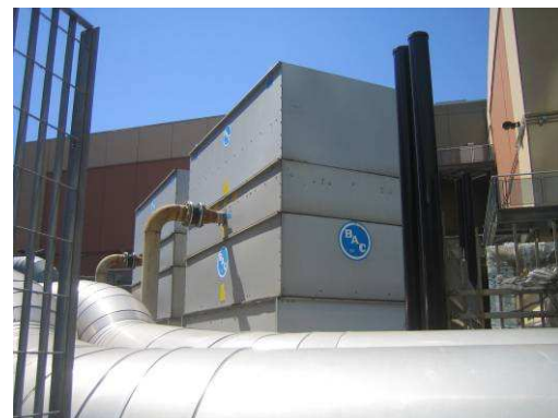
Figure – evaporative towers
