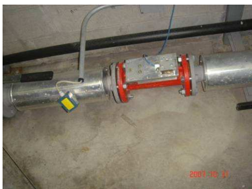
Figure – Heating consumption meter
