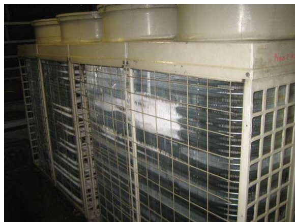
Ice formation on the external units
