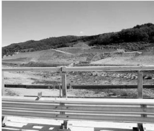
Fig. 2. Embankments and ramps in road construction project in central Italy (Oggeri, 2012)
