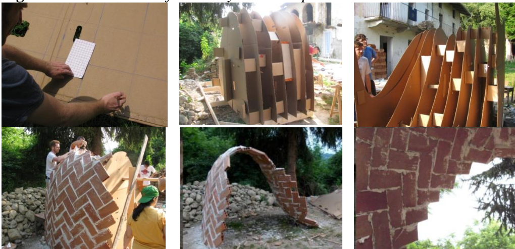
Figure 17. Sequential Steps of Formwork Construction
