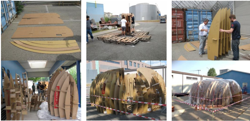
Figure 18. The Process of Final Fabrication
