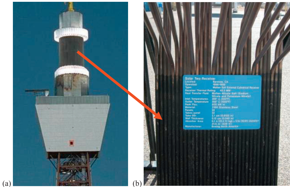
Fig. 1. (a) The Solar Two receiver. (b) Detail of one of the 24 panels of the Solar Two receiver with 32 tubes.
