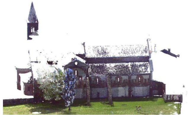
Figure 3. Coloured and merged point clouds of the north facade - image extracted from 3D Reshaper
